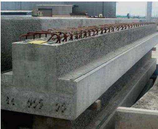
**Figure 19.** Standardisation of beams is typically on a 50 mm module, but is less restrictive, as timber or steel moulds can easily be adjusted.
