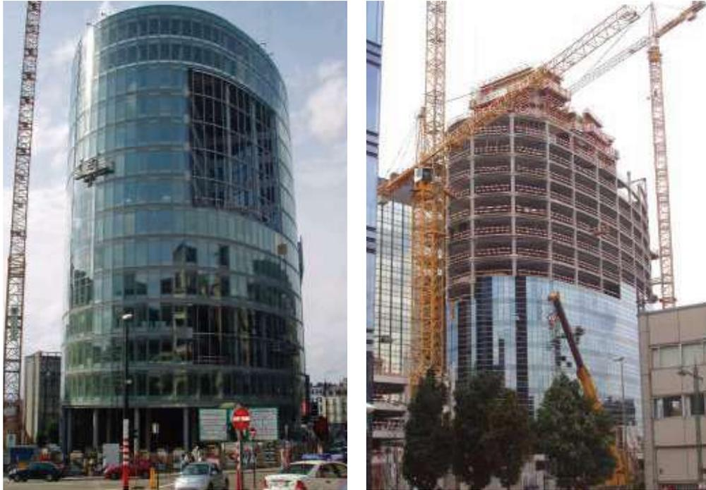
Figure 14. Oval and ellipse shaped precast concrete skeletal frames. C. Consoli, Belgium, 2008.
